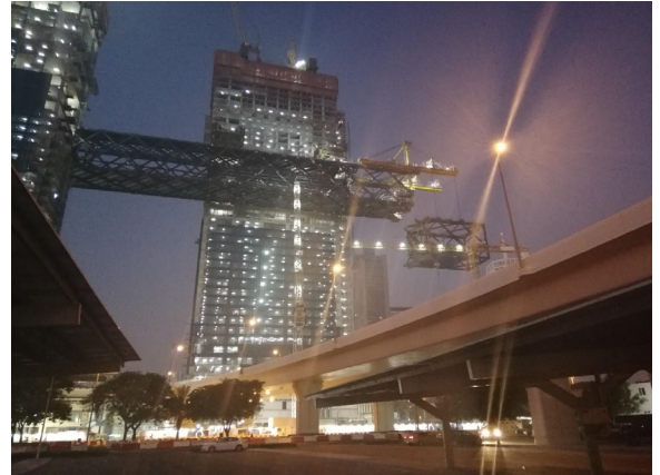
Phase 2 Lifting in progress
