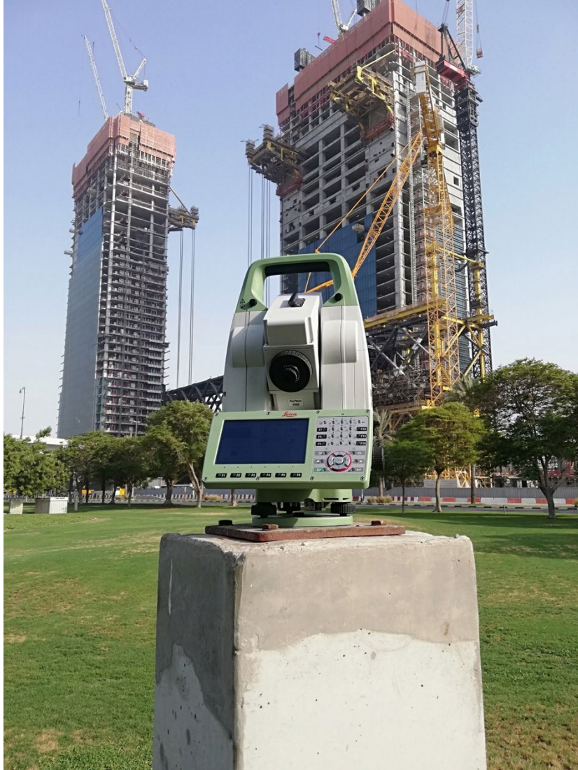
Checking the installed 3D prism targets in the gantries
