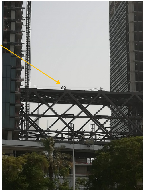
Installation of the prism targets on the Link Bridge
